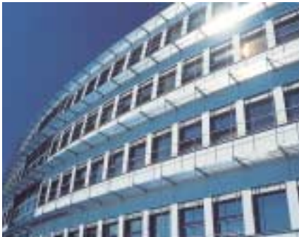
ENERGON Ulm: The administration building of the Software AG foundation is the largest office building in the world built to the passive house standard. Thermix® warm-edge spacers are built into the windows and the facade. Architects: oehler + arch kom
