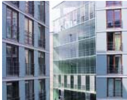
The Burse student hall of residence in Wuppertal is the largest residential building in Germany to be extensively renovated and achieve the passive house standard. Architektur Contor Müller Schlüter
