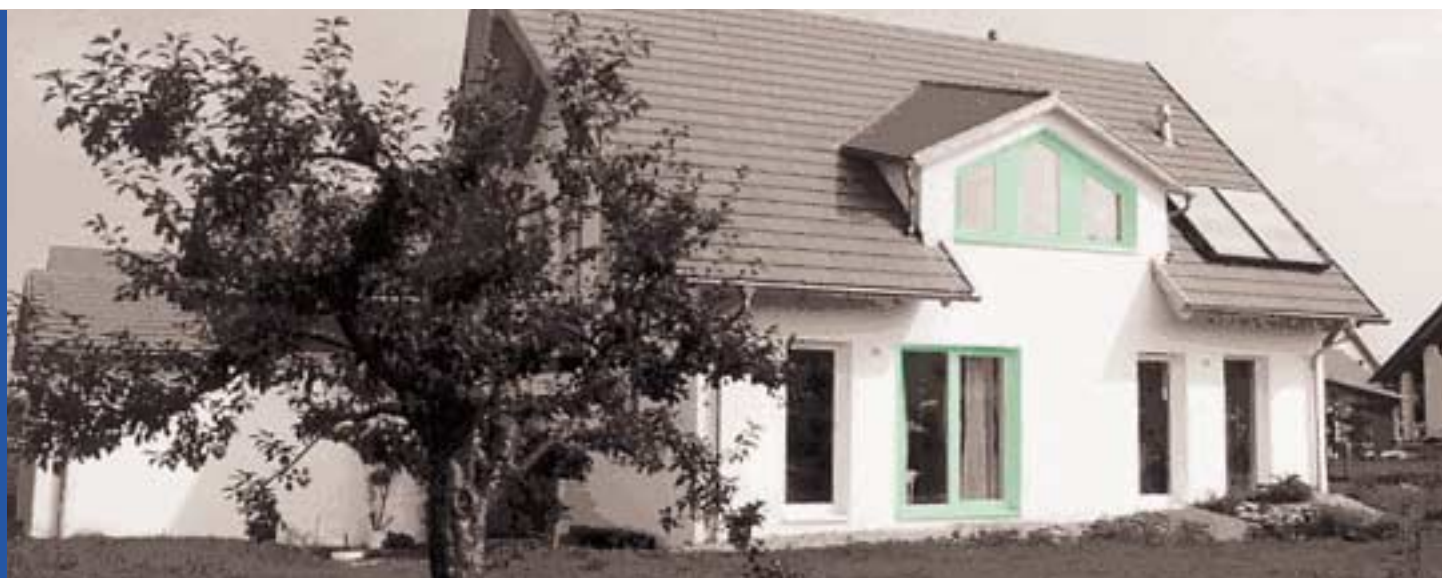
1.5-storey single-family home with 144 m 2 heated living area in low-energy building standard
